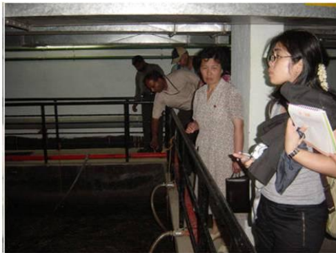
Sedimentation and aeration tanks
