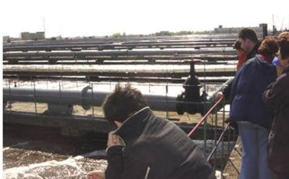
Aeration lagoons in a city sewage treatment plant (J-O Drangert)
